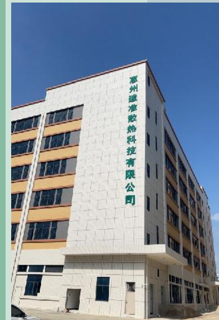
New Factory Huizhou, Guangdong Under construction
